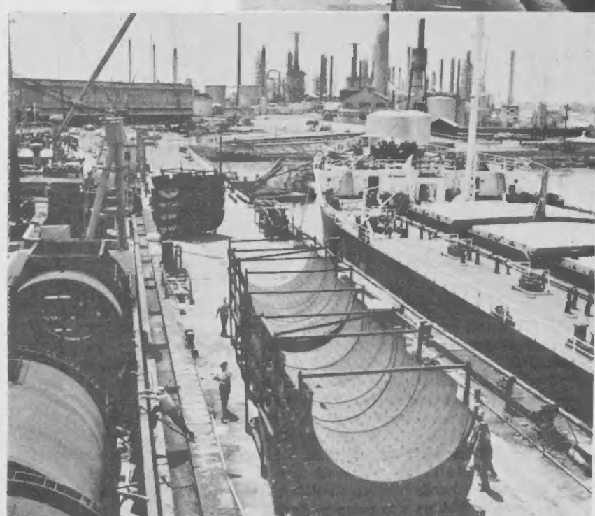
SECTIONS OF duct work, fabricated in halves in Japan, were lifted in bunches and placed on the pier. The dockside activity at No. 2 Finger Pier lends interesting patterns. SECCIONNAN DI tubo, fabricá na mitar pida na Japon, tabata worde hizá den grupo y depositá ariba waf.
